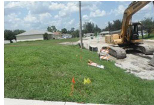
Flagged Utilities in ROW
