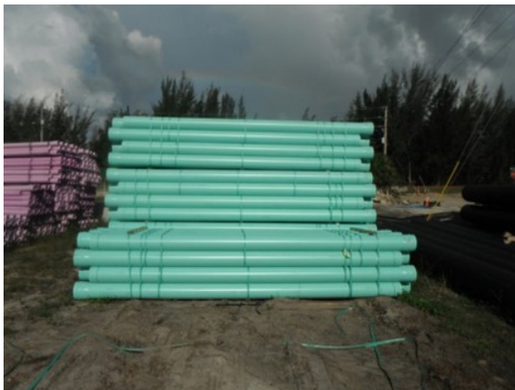
Sewer Pipes (Green Color Pipes)
