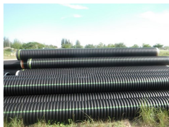
Stormwater Pipes (Black Color Pipes)
